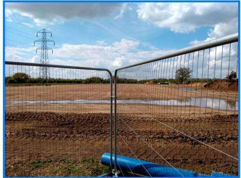
Recreational areas including football pitches under construction at St Giles Park
