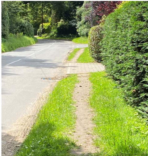
Photo 3— view looking towards Brettingham junction of mud paths created by pedestrians alongside the hedgerows of the two houses neighbouring the junction
