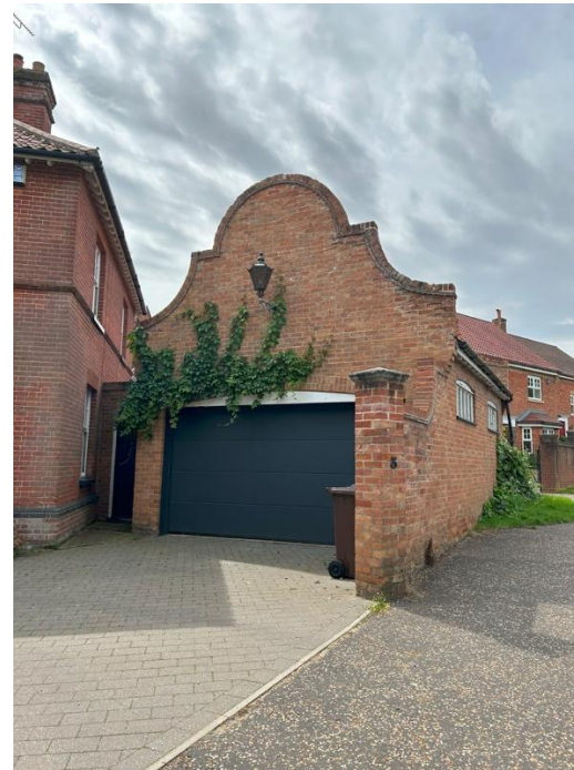
Figure 62 Garage and side parking along Newmarket Road
