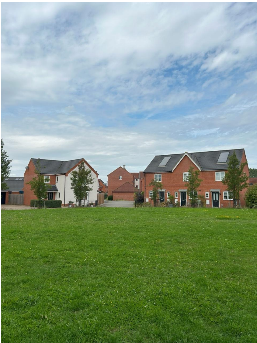
Figure 69 Examples of solar panels on residential dwellings within St Giles Park
