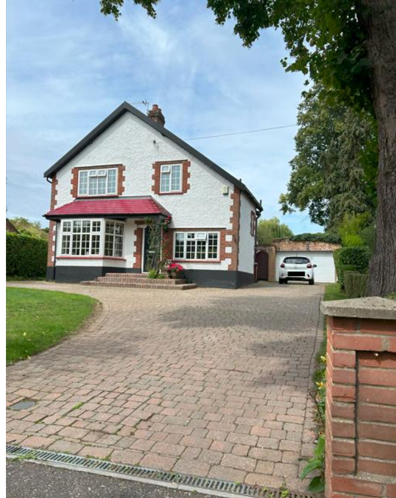
Figure 45 Example of residential dwellings set back from the highway with large front driveways along Intwood Road
