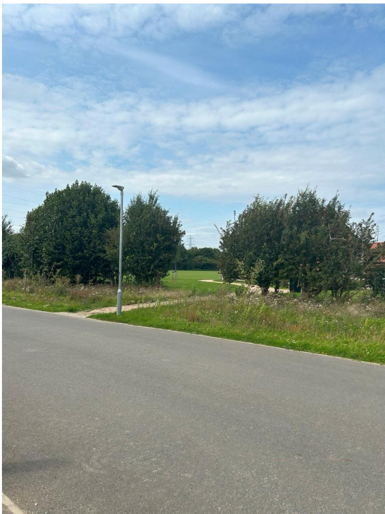
Figure 91 Examples of street lighting at the entrance of green open space within the St Giles Park development
