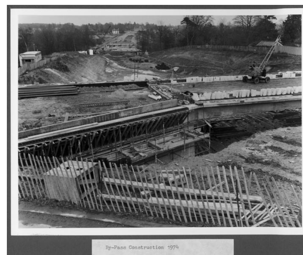
Figure 11 Thickthorn bypass construction in 1974 (Source: Cringleford Historical Society)
