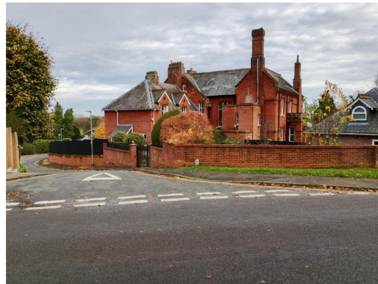
Figure 102 Oakland House, Colney Lane
