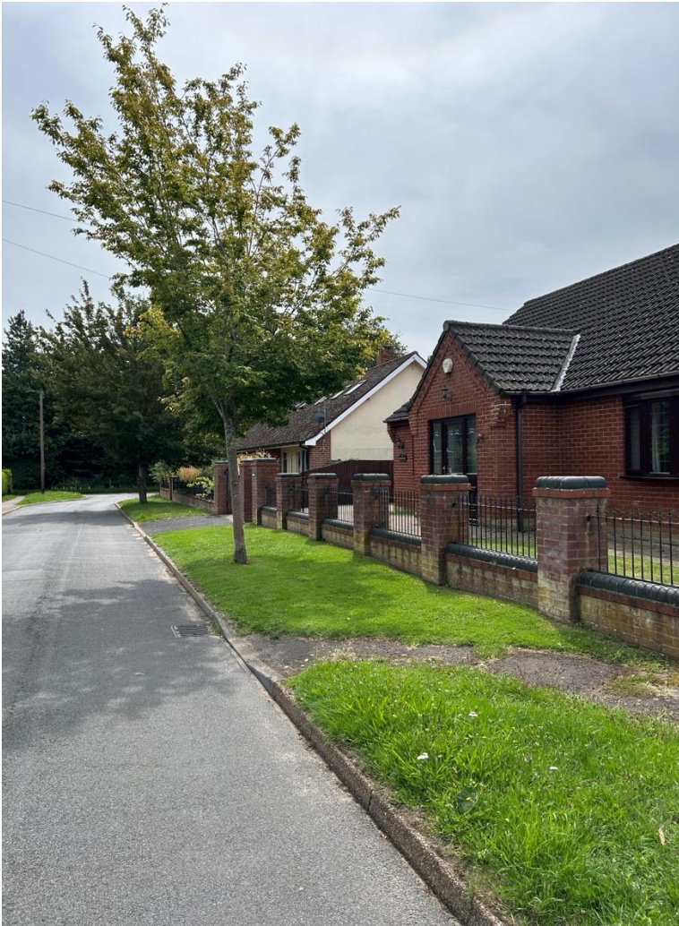
Figure 112 Example of the boundary treatments within CA2
