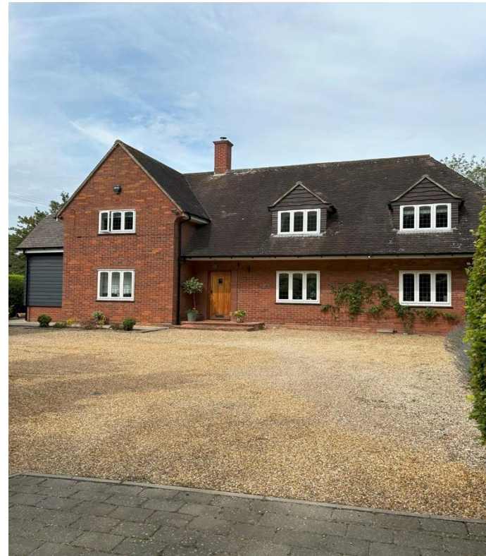
Figure 60 Ample front parking along Intwood Road
