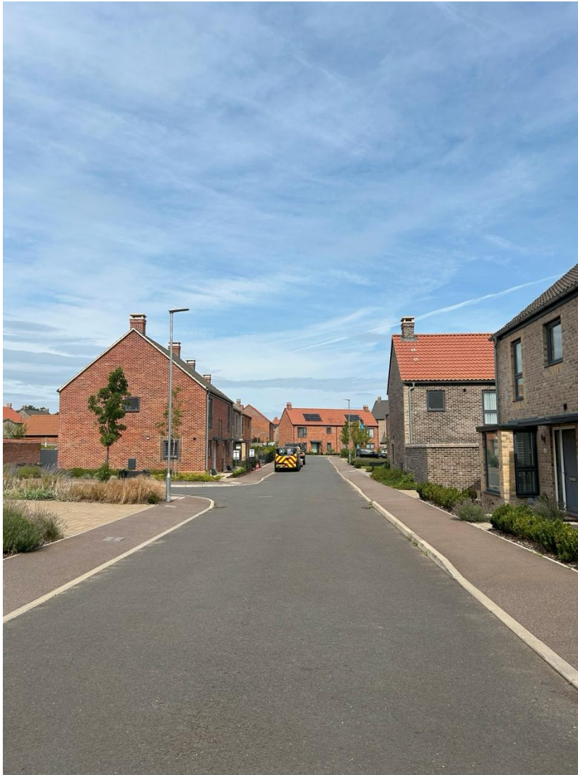
Figure 48 Examples of new residential dwellings following a linear form close to the highway along Shenkwyn Rd within St Giles Park development
